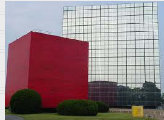
Public Safety Headquarters Baltimore County
