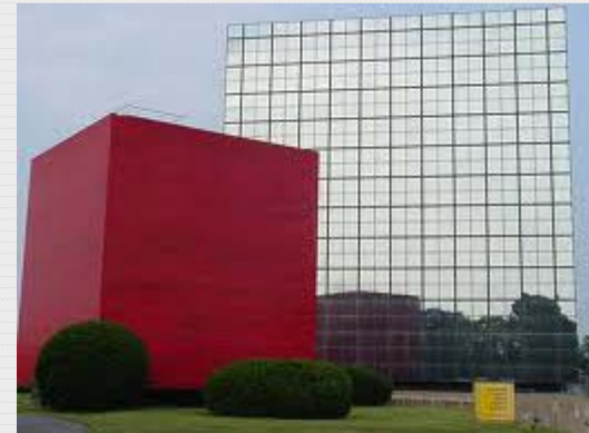
Public Safety Headquarters Baltimore County
